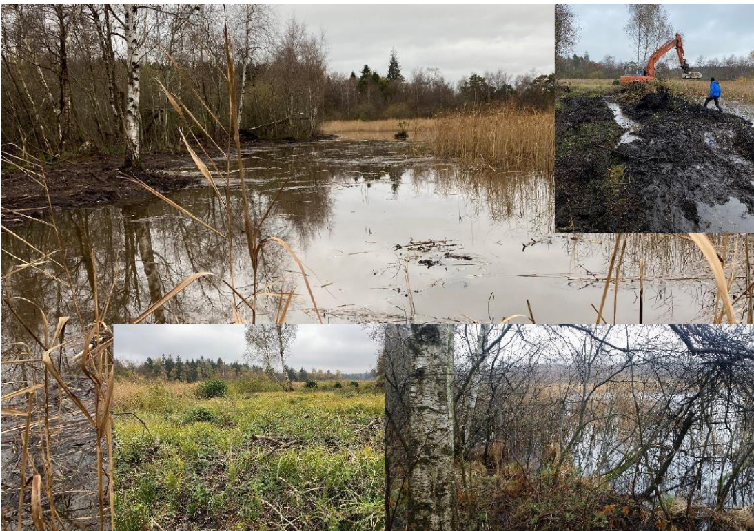
Figure 6 Increasing the area with open shallow water during implementation of C2. Photo: N.Damm
